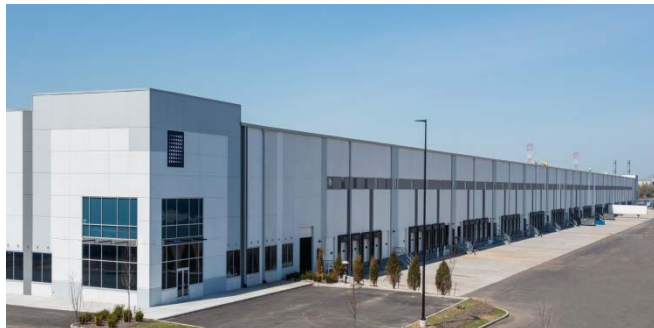
586 Gulf Avenue, Staten Island, NY
