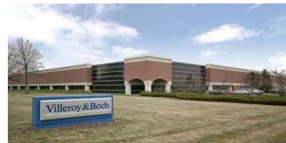
3 South Middlesex Avenue, Monroe, NJ
